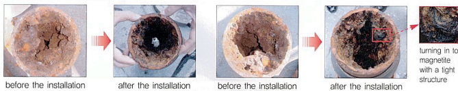
before the installation
