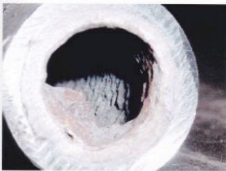
Before installing ISB ( Scale in pipe )
