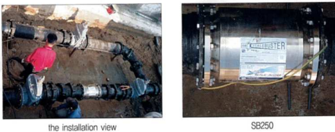
Pipe annuli-buried in 2002
