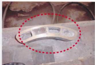
Before installing ISB ( holder in furnace )
