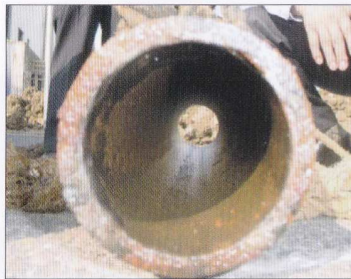
3 years after the installation (October 26, 2005)
