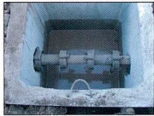
confirming installment sites
