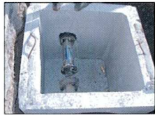
Installing Scale-Buster/ installing pipe annuli
