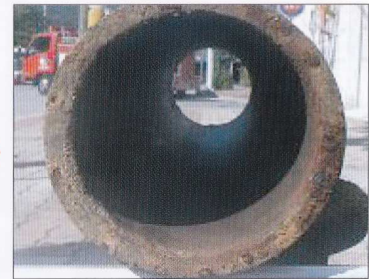
5 years after the installation (October 4, 2007)
